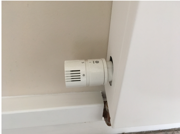
The Thermostatic valve is graduated from 1 to 5, with 1 being the frost setting.
